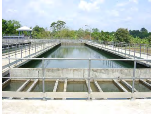
Kadana water treatment plant
