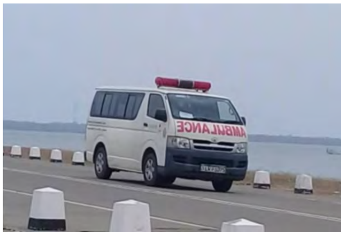
Photo 1: Emergency ambulance transportation to the east-bank side of the bridge became easy
