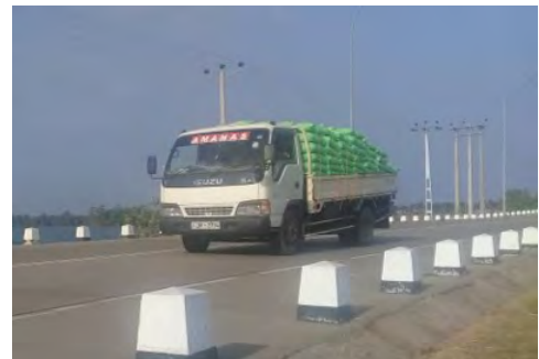
Photo 2: The opening of the bridge contributed to reducing truck delivery time and cost
