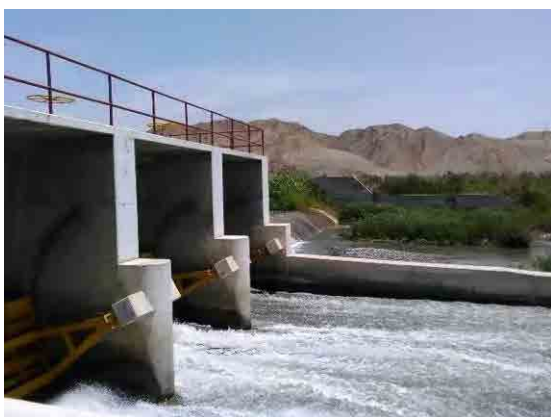
Headwork (Lima Region)
