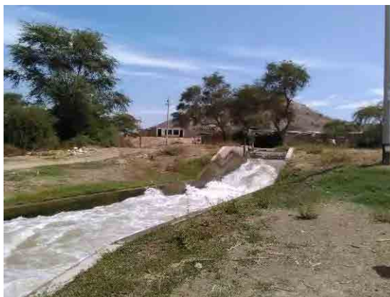
Rehabilitated canal (Lambayeque Region)
