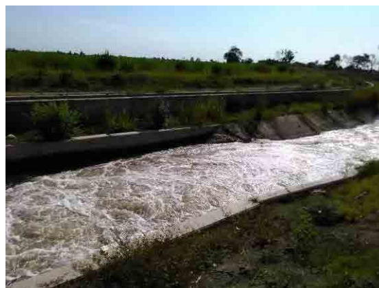
A rehabilitated canal (Lambayeque Region)
