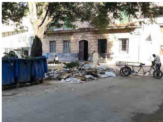
Construction wastes illegally disposed on the street
