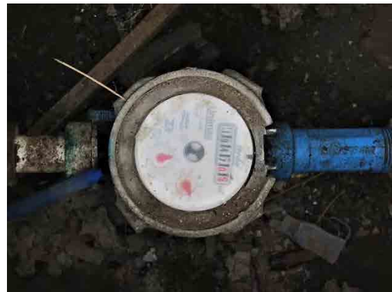
(Left) Street where water supply and sewerage rehabilitation were made (Right) Newly installed water meter (outside of the Project scope)
