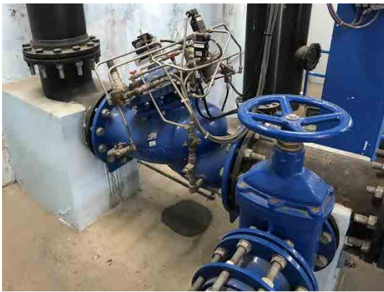
(Left) Valves at a distribution tank connected to SCADA (Right) SCADA control room (SEDAPAL headquarters)
