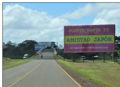
Access road and the Bridge
