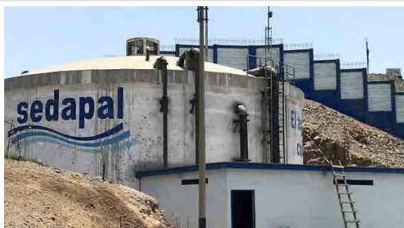
Distribution tank rehabilitated by the Project
