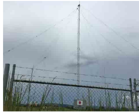
Short Wave Antenna Mast
