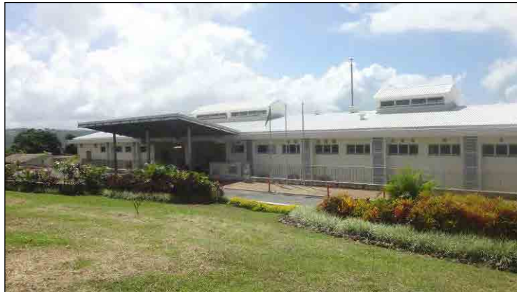
New Hospital Constructed in the project
