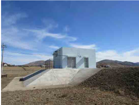
One of the wells constructed through this project
