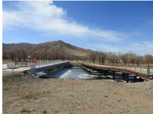
Maintenance bridge (left) and temporary bridge
