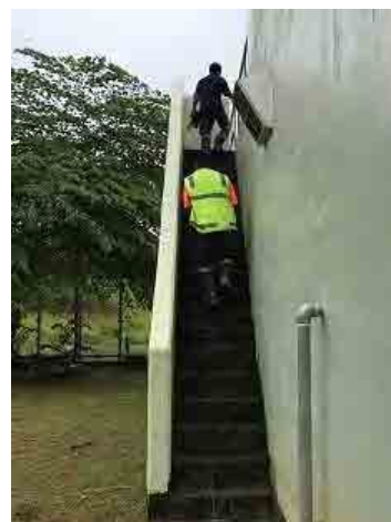
Stairs for chlorine facility (Tasahe Pump Station)
