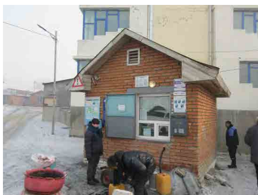
Water supply at a kiosk (at the time of ex-post evaluation)
