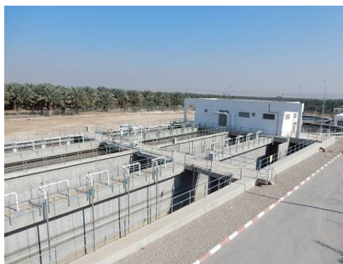
Constructed Waste Water Treatment Facility
