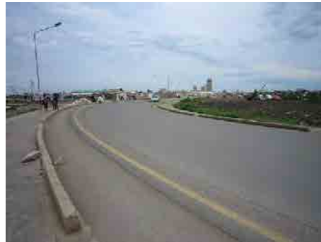
Part of constructed road
