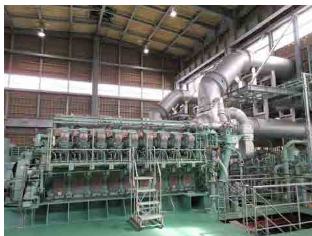
Generator Installed in this Project
