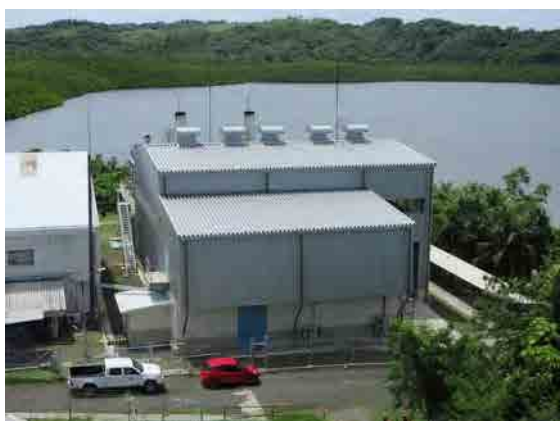
Panoramic View of the Power House
