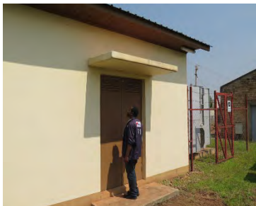
Ngoma Distribution Post (Huye distribution network)
