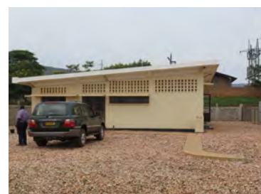
Substation Building (Rwinkwavu)
