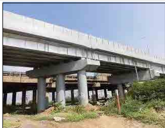
Athipattu Rail Over Bridge Built as Small Infrastructure Project
