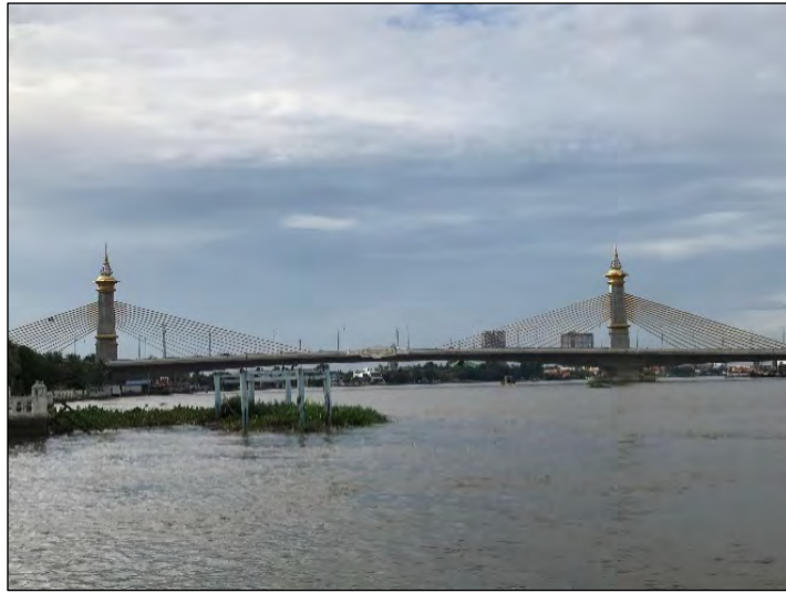
Maha Chesadabodindranusorn Bridge constructed by this project
