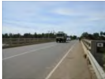
MEBON Bridge (BR-8 Bridge) after reconstruction
