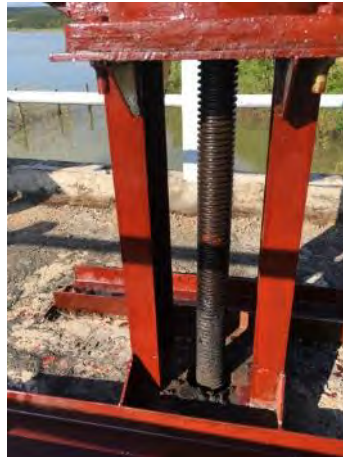
Irrigation subproject. Reservoir and dam head works (Kon Tum Province)
