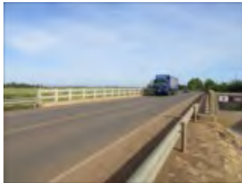
KBAL BOEUNG Bridge (BR-4 Bridge) after reconstruction
