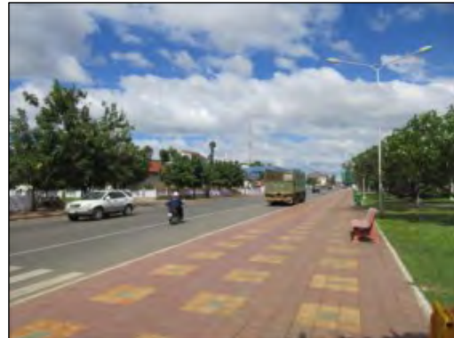
Vehicles passing over the national Road No. 5 after improvement.
