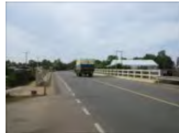
ROM LECH Bridge (Clv-2 Bridge) after reconstruction
