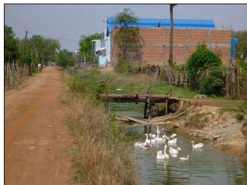
The canal rehabilitated by this Project
