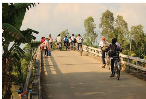
With the construction of a bridge directly connected to the school, it has become possible to go to the school by bicycle rather than small boat (Soc Trang Province)
