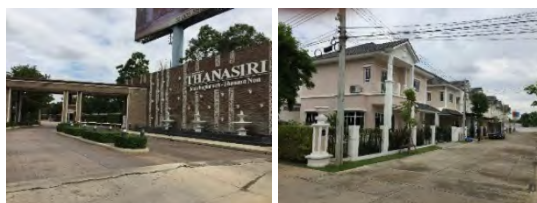
New Housing Project (Thanasiri)
