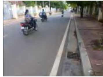
Installed Drainage System (in Kampong Chhnang City)
