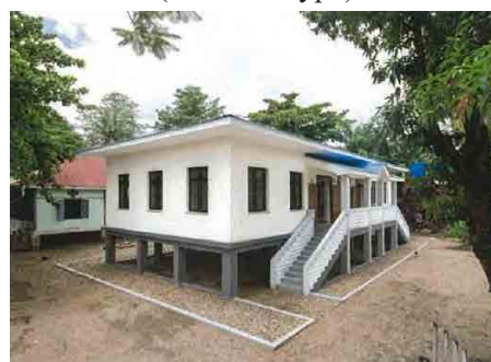
Appearance of a newly-constructed RHC (Raised-floor type)
