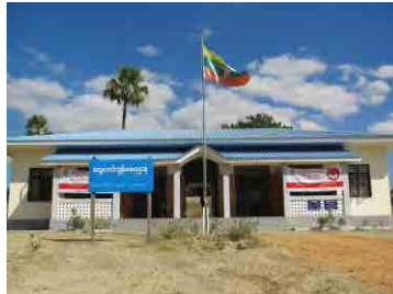
Newly-constructed Lat Seil RHC (at Ex-post Evaluation)
