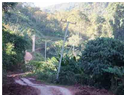
Figure 3: Slanting Pole
