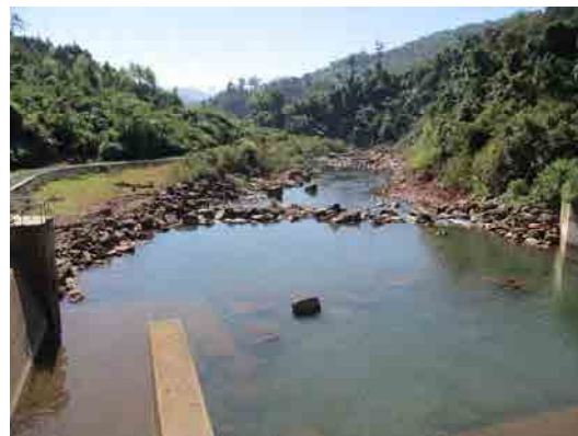
Figure 2: Washed out Concrete Blocks
