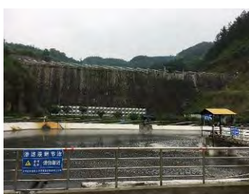
Leachate treatment facility at a waste treatment and disposal facility
