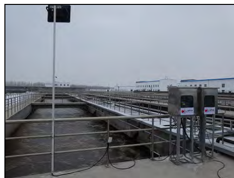
Kuitun Sewage Treatment Plant (activated sludge tank)
