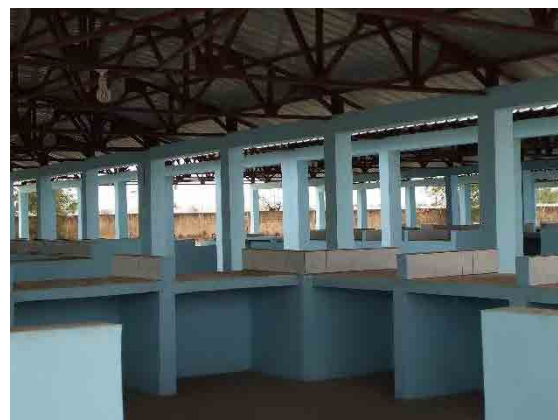
Hangar for fresh fish retailers (MCPB)
