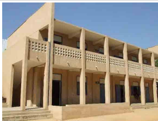
Classrooms constructed by the project (Cheikh Awa Balla Mbacké Secondary School, Dakar Region)
