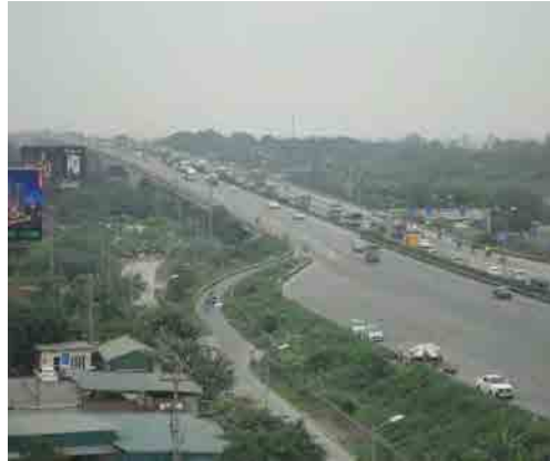
Red River Bridge
