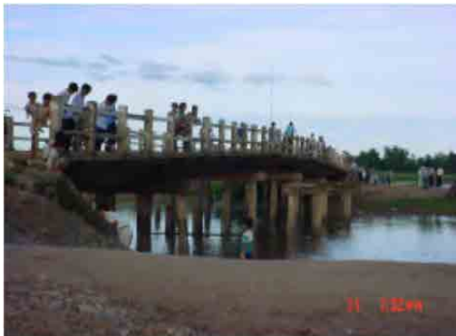
Quynh Bang Bridge At the time of Planning (2001)
