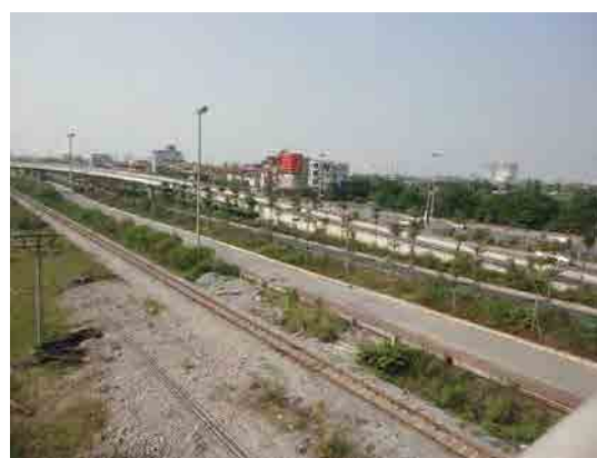
A Part of Clover Leaf Interchange and Rail Road after Realignment
