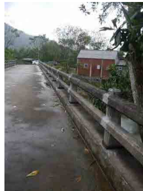
Khe Duong Bridge with repaired guardrails
