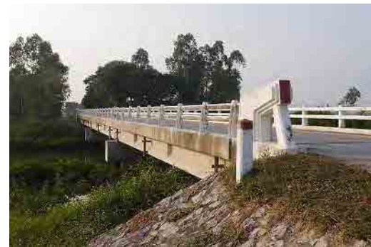
Quynh Bang Bridge At the time of Ex-post Evaluation (2017)
