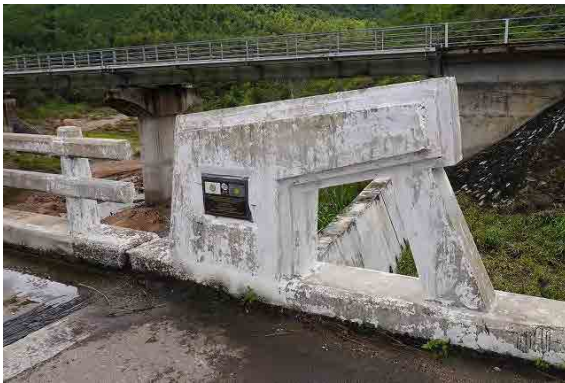
Tra O Bridge with repainting
