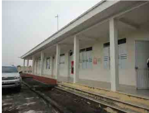
Building of a substation constructed in this project (Yen My Substation, Hung Yen province)
