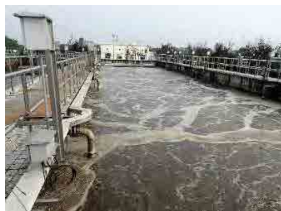
Songya Treatment Plant in Mianyang city
