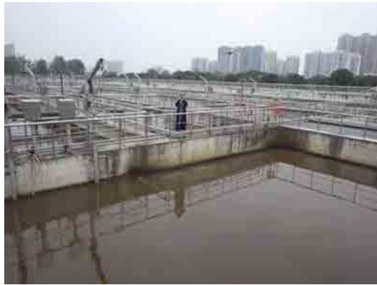
Aeration tank at the North-area Wastewater Treatment Plant (The improved A 2 O process was adopted)
