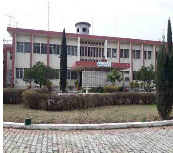
Faqirabad Transmitting Station
