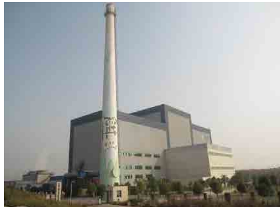
The newly-built household solid waste incineration plant
