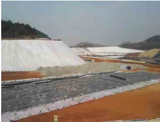
Landfill facility constructed under the Project (Huarong)
