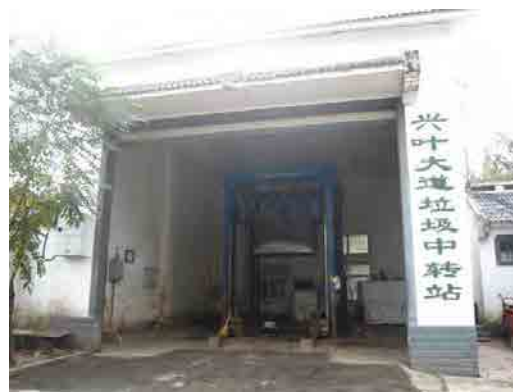
Transfer station set up for the current project (Yè jí)
