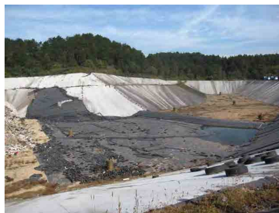
Landfill constructed for the current project (Huoshan)
