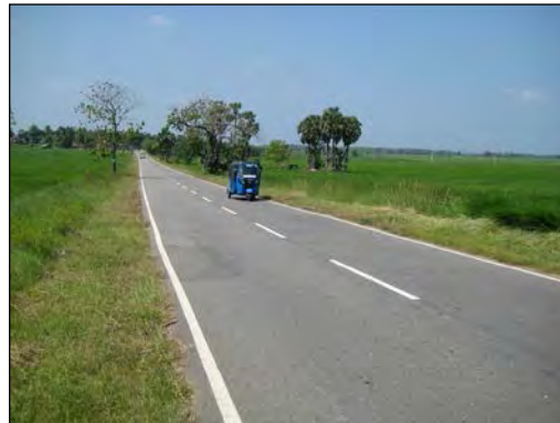
National Road (Deegavapi Temple Road) in Ampara District, Eastern Province rehabilitated by the project
