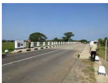
Mundeni Bridge (No.2 Bridge) after reconstruction
