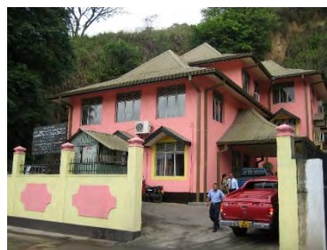
Head Office of PRDA, Central Province renovated by the Project
