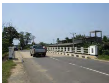
Mahaoya Athuganga Bridge (No.1 Bridge) after reconstruction
