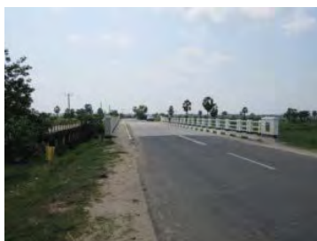
Chenkalady Bridge (No.4 Bridge) after reconstruction
