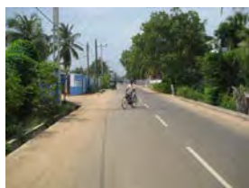
Provincial Road in Batticaloa District, Eastern Province (Beach Road)
