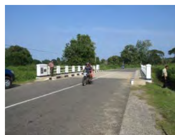
Pulavady Bridge (No.3 Bridge) after reconstruction
