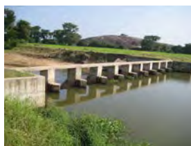
Anicut in Ampara District, Eastern Province (Sagama Irrigation Scheme)
