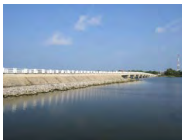
Panichchankeni Causeway and Bridge (No.5 Bridge) after reconstruction
