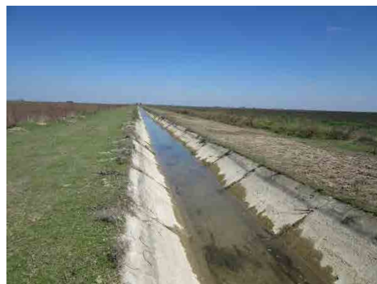
Irrigation Canal Rehabilitated in This Project (Djizzak Province)
