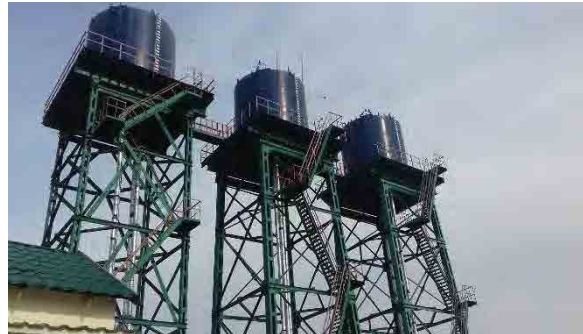
Elevated Water Tank Constructed in This Project
