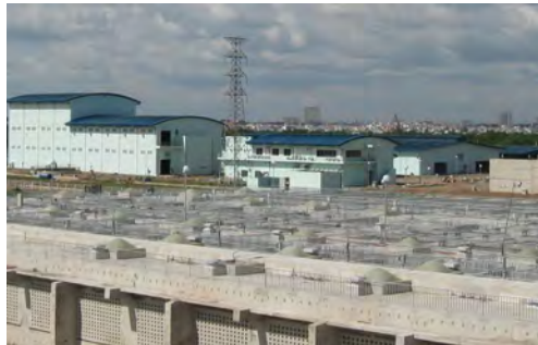
Binh Hung Wastewater Treatment Plant
