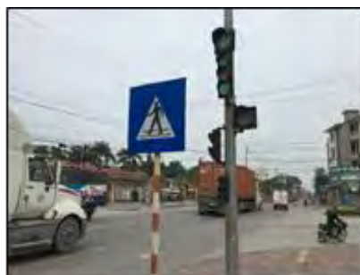
The Installed Traffic Sign and Light
