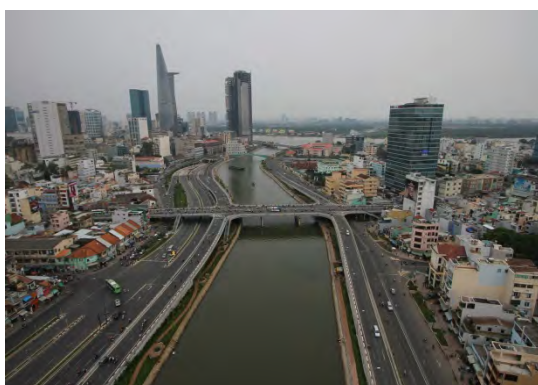
Photo 1: Road Developed by this Project (left side) (Photo provided by construction management consultant)
