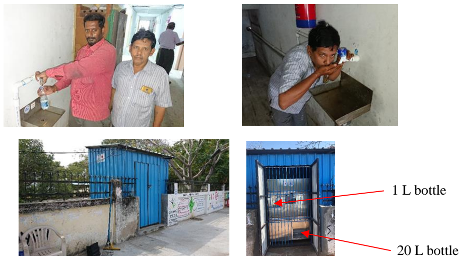
Figure 9 Drinking Water Dispensation Points & Drinking Water ATM
