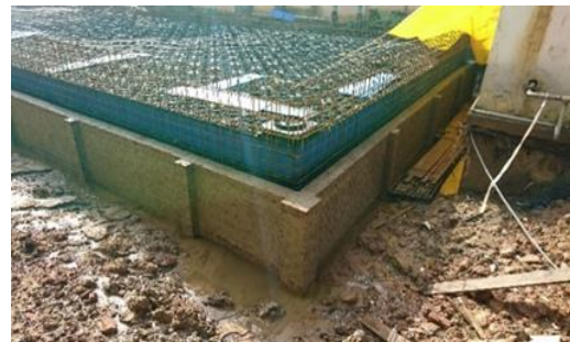
Sidewall Construction
