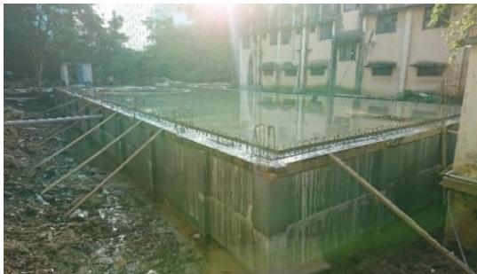
Sidewall & Slab Concrete
