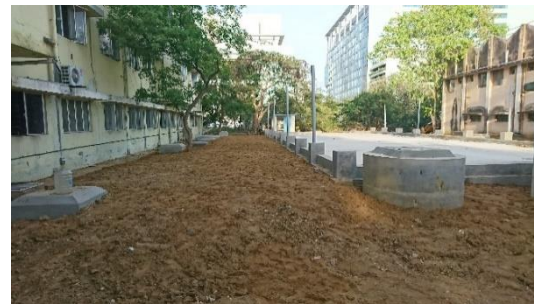
Backfilling & Ground Leveling Work
