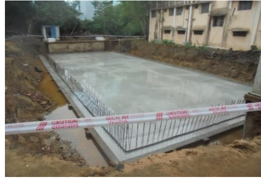
Base concrete & Rebar Work for Sidewall
