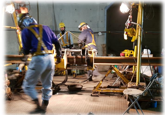
Gas Pressure Welding
