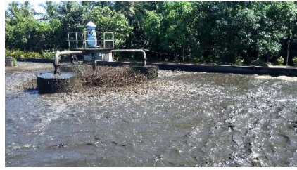
Photo 4.1.2 C1 Aeration Tank
