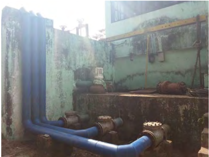
No.4 Pump Pit (Raw Water Pit)
