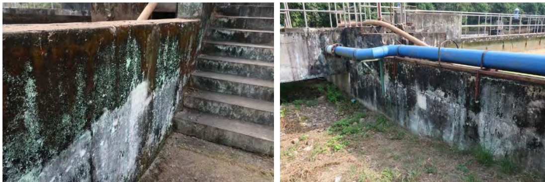
Photo 1: Concrete Surface of Reactor in C1 WWTP
