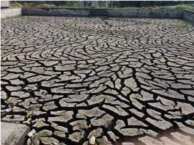
No. 12 Sludge Drying Bed
