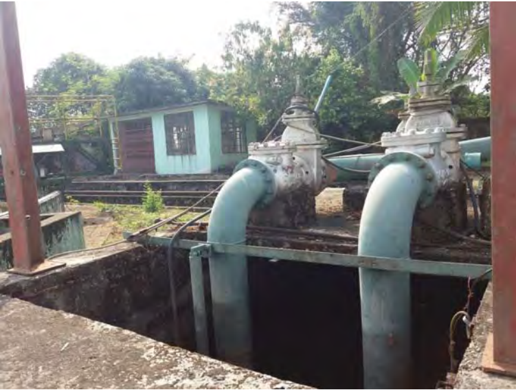
No.10 Return Sludge Pump Pit
