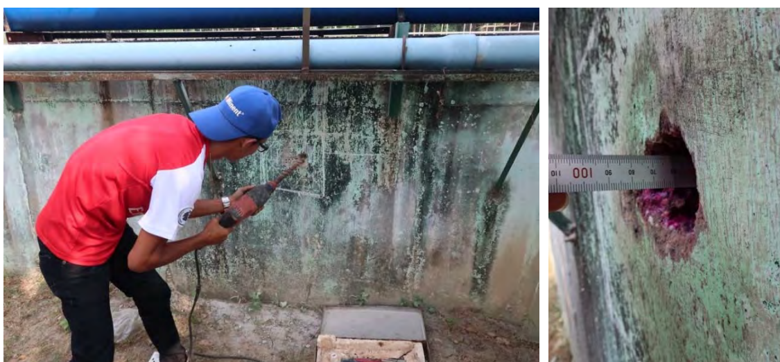
Photo 2: Concrete Chipping Survey (Reactor of C1 WWTP)
