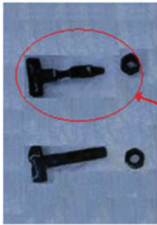
Case of corrosion on the bolts
