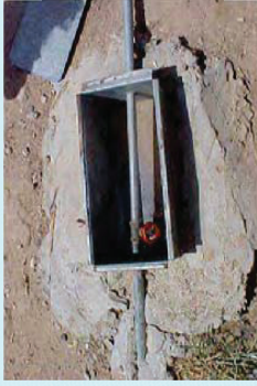
Remove the water meter
