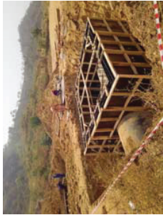
Chamber Construction for Bulk Meters (Activity 1-1)
