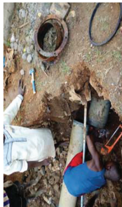
MAINTENANCE OF LEAKAGES ON 300MM DIA UPVC PIPE
