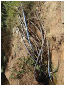
Service Pipes to Villages in Jabi
