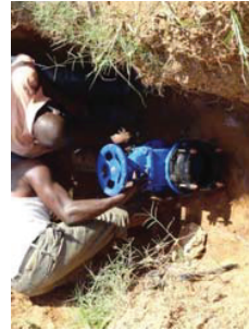
Installation of Isolating Valve (Activity 2-7)
