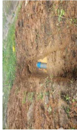
MAINTENANCE OF LEAKAGES ON 300MM DIA UPVC PIPE
