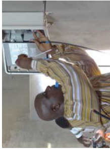
Installation of Zonal Meter's Main Unit (Ultrasonic Flowmeter)
