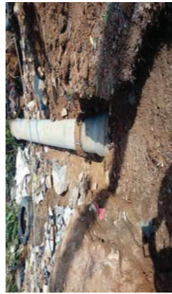
MAINTENANCE OF LEAKAGES ON 300MM DIA UPVC PIPE
