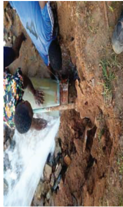
MAINTENANCE OF LEAKAGES ON 300MM DIA UPVC PIPE
