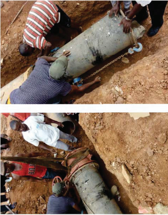
CONSTRUCTION WORKS ON THE FAILED CONTROL VALVES AT NYANYAN WATER SUPPLY
