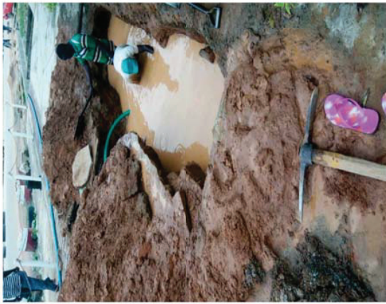
CONSTRUCTION WORKS ON BURST PIPE AT CENTRAL AREA & WUSE
