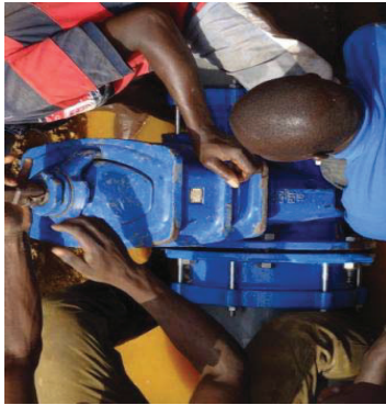
Install of New Valve
