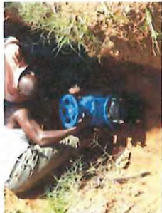
Installation of Isolating Valve (Activity 2-7)
