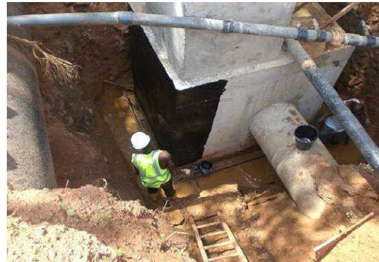
Chamber Construction at Tank Kubwa
