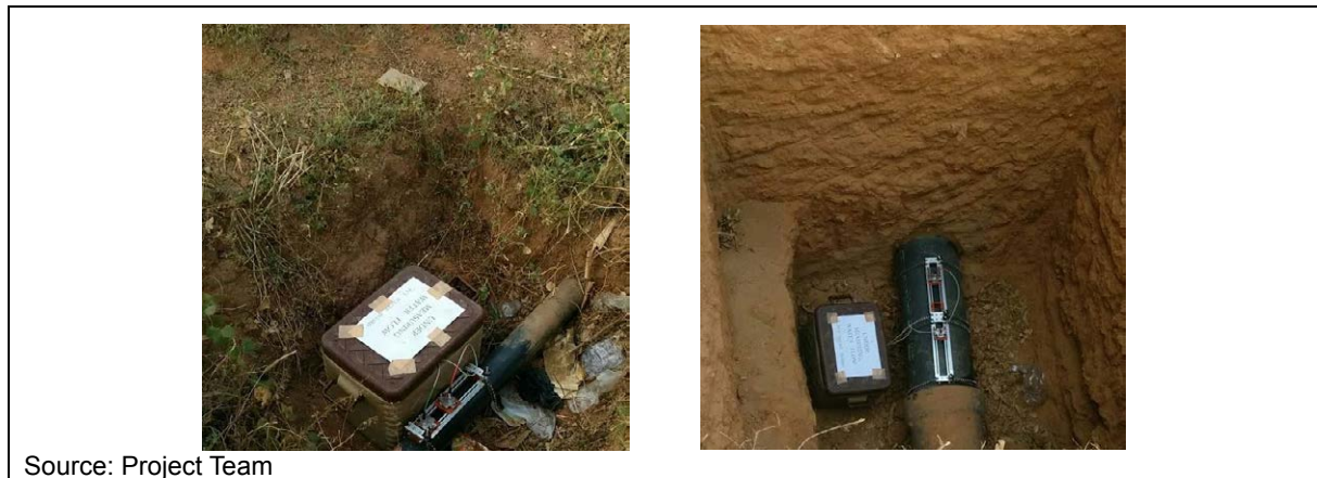
Figure 3.2-34: Installation on Pipeline, Ultrasonic Flowmeter
