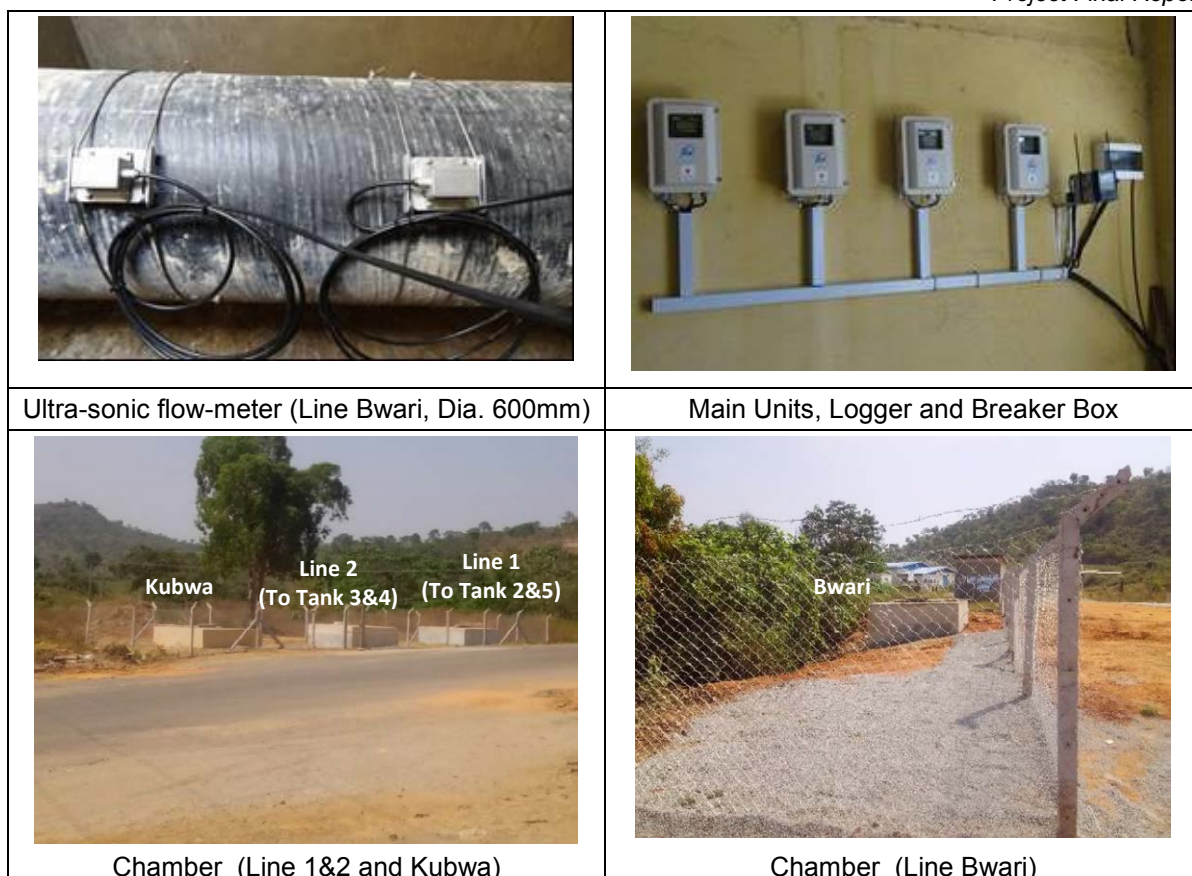
Figure 3.2-3: Bulk Flow-meters, Chambers and Cables
