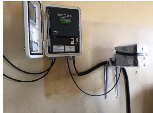
Zonal Meter and Logger at Tank Airport
