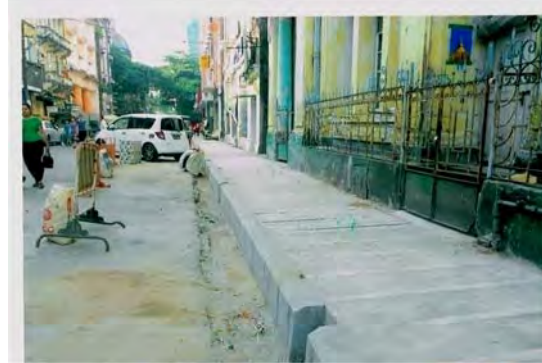
Completed Drainage Culvert below Walkway
