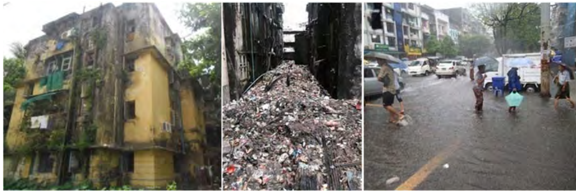
Old Building with Weak Infrastructure
