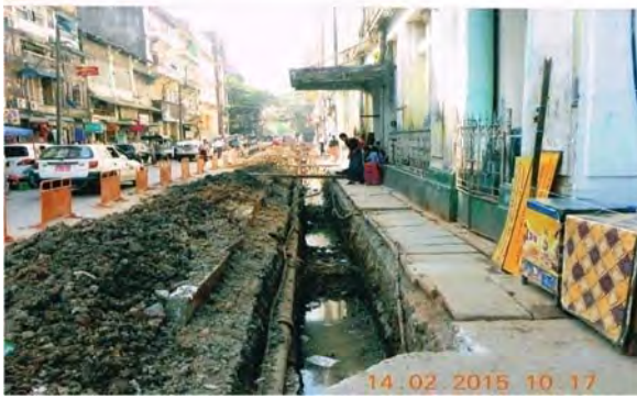
Under Construction of Drainage Culvert below Walkway
