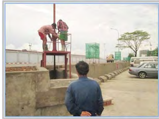
(b) Drainage Sluice Gate on Outlet at Yangon River (Strand Rd.)
