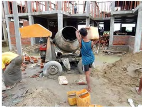
Side-mixing of concrete
