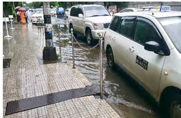
(c) A Paddle Immediately in Front of Drainage Inlet Beside a Major Highway
