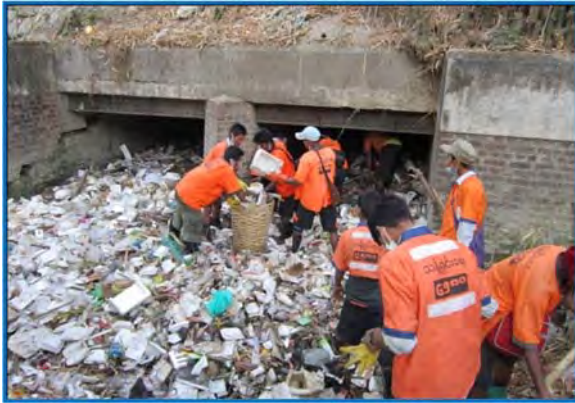
(a) Removal of Garbage in front of Drainage Outlet
