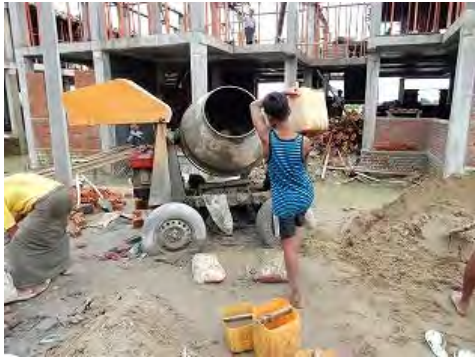
Figure 3.3.4: Side-mixed concrete
