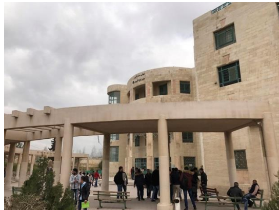
School Building of Al-Balqa Polytech University
