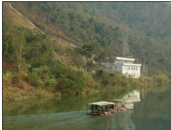
Hydropower Plant in Nghe An Province
