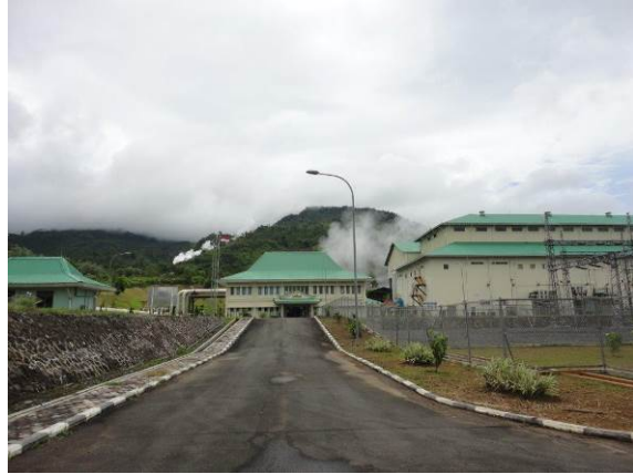
Ulubelu Geothermal Power Plant
