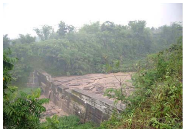
Arrested Debris Flow by Sabo Dam at Krasak River (Source: Material provided by Executing Agency)
