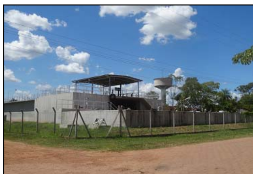
Concepcion Water Treatment Plant
