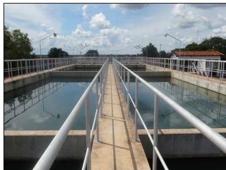
Concepcion Water Treatment Plant: Chemical Sedimentation Tank
