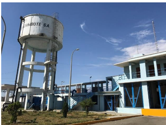
Distribution Reservoir (Chimbote)
