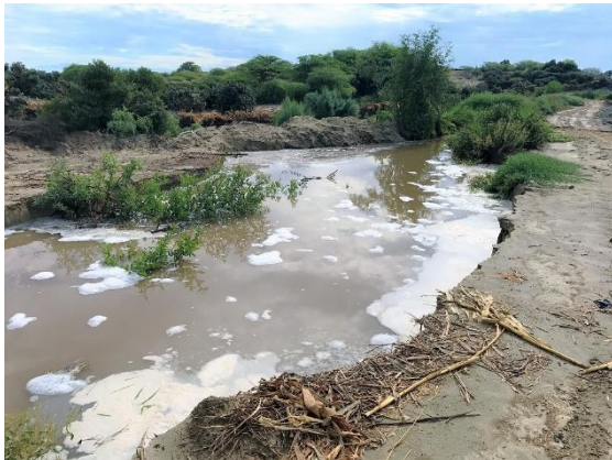
Extension of outlet channel for El Indio STP (Piura)
