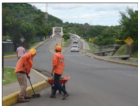
FOMAV workers conducting cleaning work near Tecolostote Bridge
