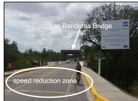
Speed reduction zone at Las Banderas Bridge (towards El Rama)
