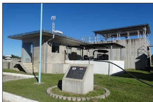
Pilar Water Treatment Plant
