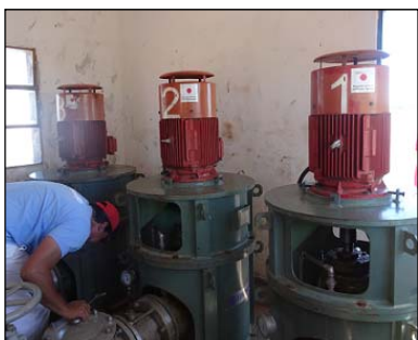
Pilar Water Treatment Plant: Inspecting the water intake pump
