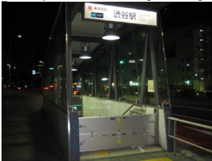
Photo: Examples of water stops installed
