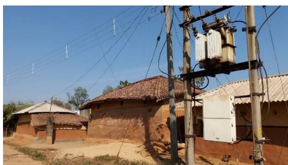
Figure 2: Settlement in the Project Site
