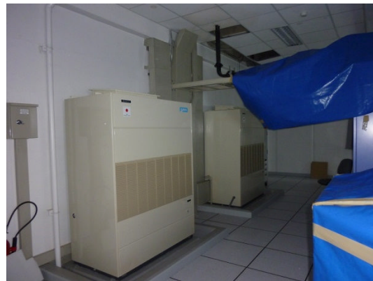
Photo 2: Water leakage sometimes occur from cracks in the ceiling caused by typhoon Nock-Ten
