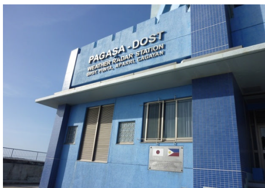
Photo 3: Metrological Radar Tower at Aparri
