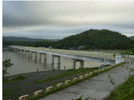
Constructed Umiray Bridge and Access Road
