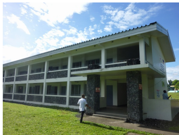
Schools Designated as Evacuation Shelters Developed under This Project (Sto. Domingo Central Elementary School)
