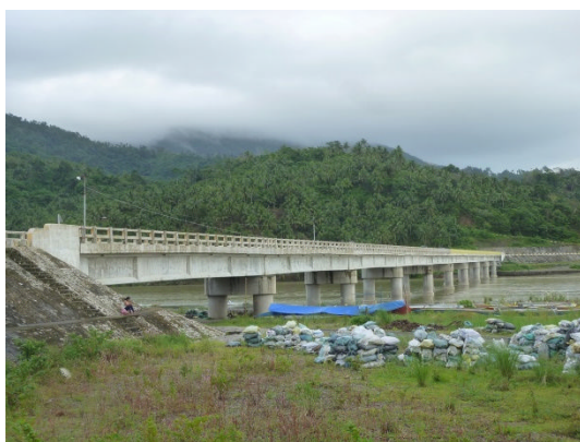
Photo 1: Constructed Umiray Bridge
