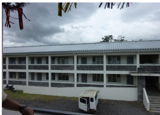
Photo 1: Polangui North Central Elementary School
