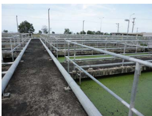
Waste Water Treatment Plant
