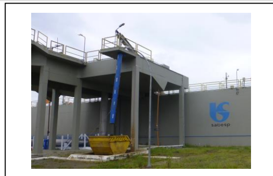
A new wastewater treatment plant in Itanhaém
