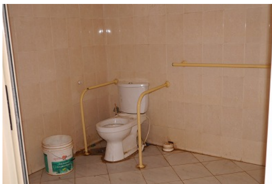
Toilet for persons with disabilities constructed by the project
