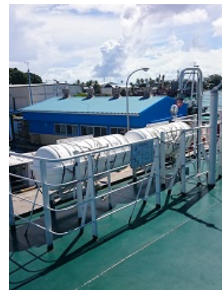
Photo 2. Inflatable life rafts installed in a vessel.
