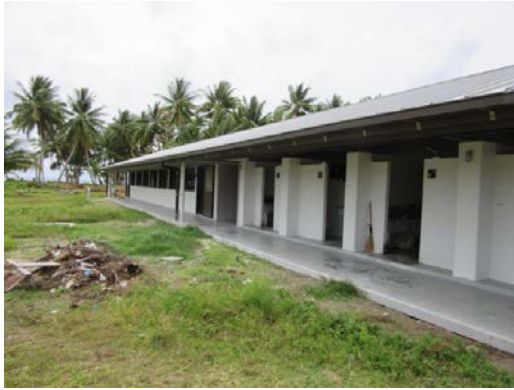
Girls' Dormitory Newly Constructed
