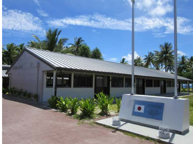
General classroom building constructed in this project
