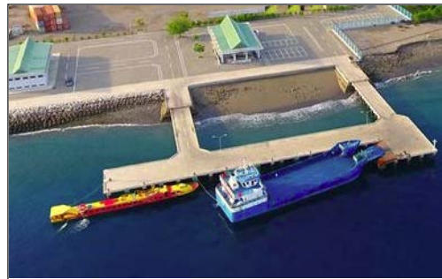
Rehabilitated Oecusse Port
