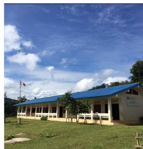
Donchan Primary school built under this Project (Sekong, Lamam)
