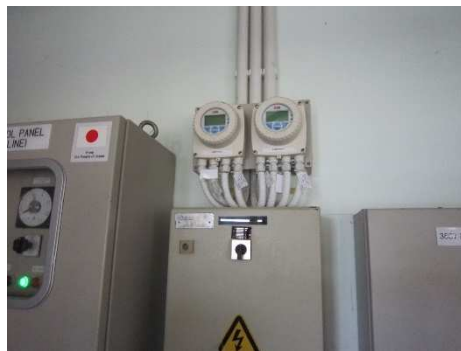
Water flow monitoring system (Left) and the meters for measuring the volume of the supplied water (Right)
