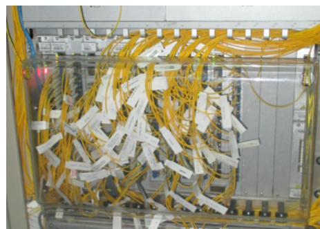
At the ex-post evaluation: Destinations of the cables can be identified easily as there are labels and the cables are bundled as needed. (The photo was taken by the external evaluator)
