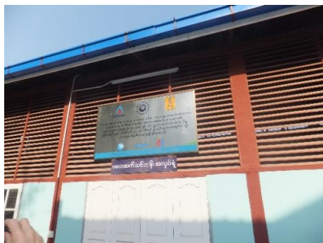
Workshop renovated for Welding department
