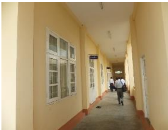
Corridor of workshop
