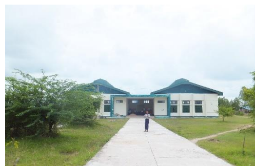
Workshop (Mechanical Engineering, Civil Engineering)
