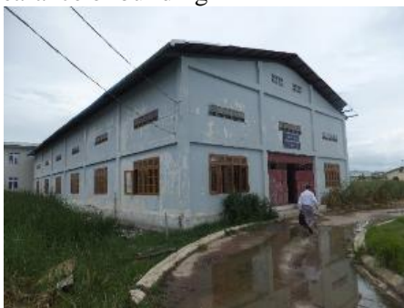
Workshop (New training ridge at behind)
