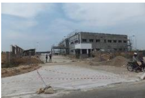
Vocational training center by Reinforced Concrete under construction
