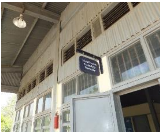
Metal Workshop 入口周り(鉄骨造+波板鉄板)
