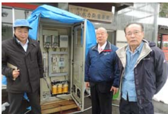
Inspection before Shipment
