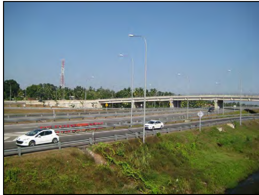
Southern Expressway near the Kottawa Interchange
