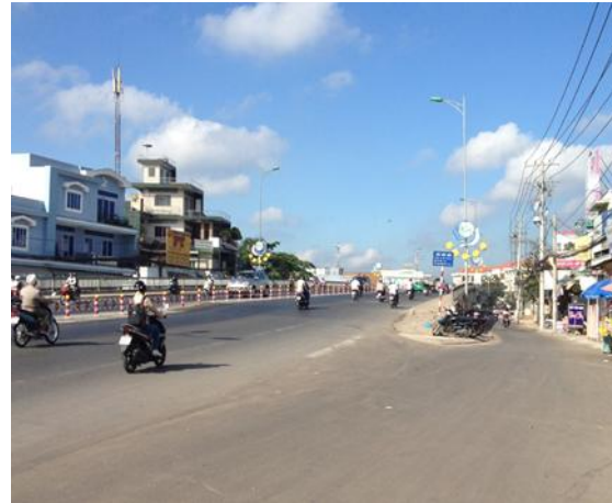
A View of Cai Rang Bridge
