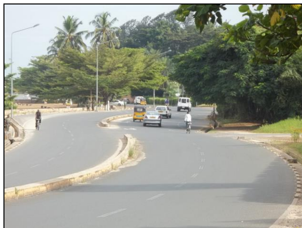
A Road Section Improved in this Project (Avenue de la Plage)
